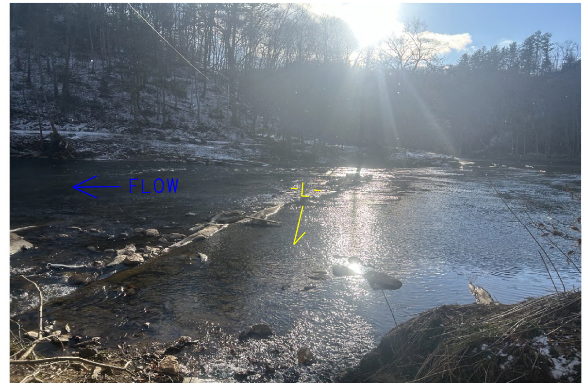
PHOTO #2: BENT NO. 3 OF NEW BRIDGE ALIGNMENT LOOKING SOUTHWEST (DOWNSTATION).
