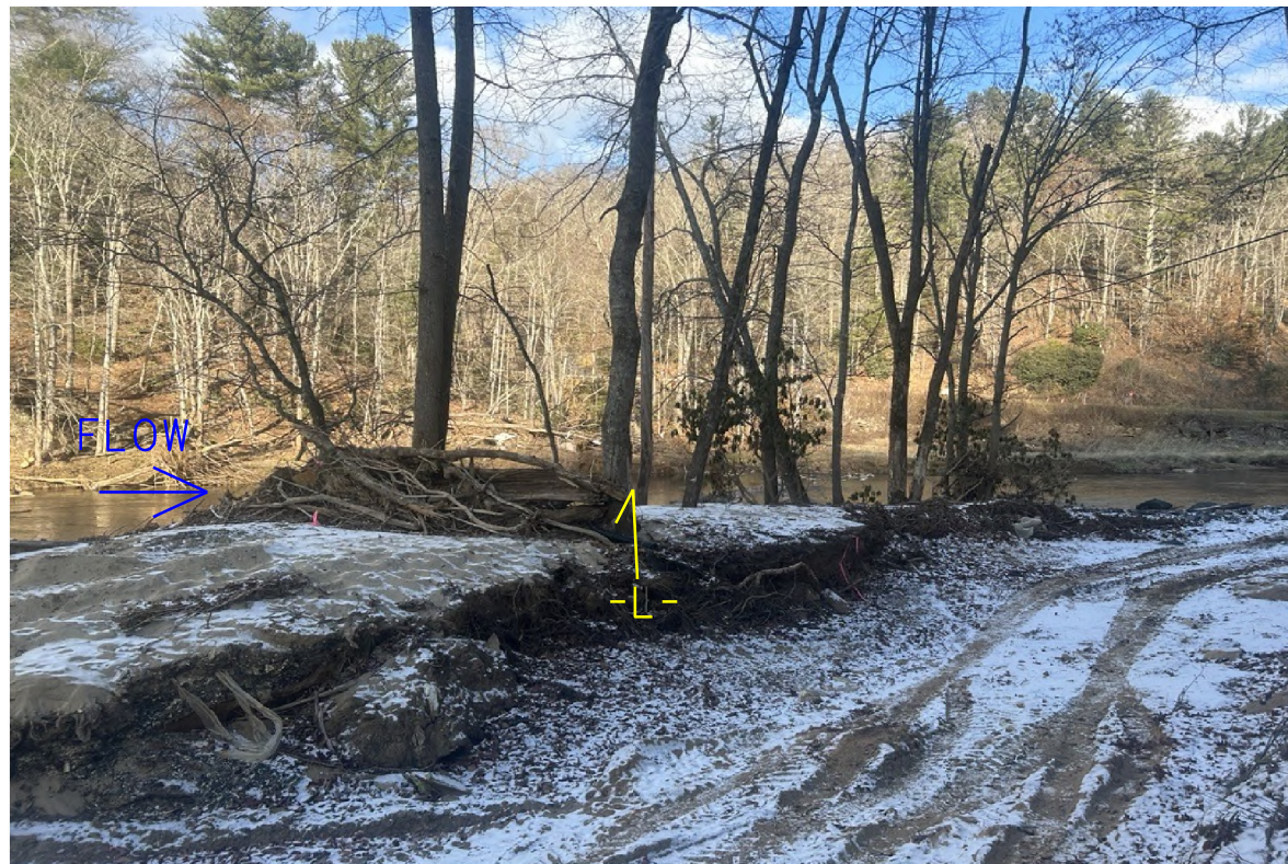
PHOTO #1: END BENT NO. 1 OF NEW BRIDGE ALIGNMENT LOOKING NORTHEAST (UPSTATION).
